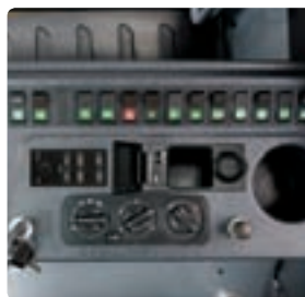
Concentrated switch panel
